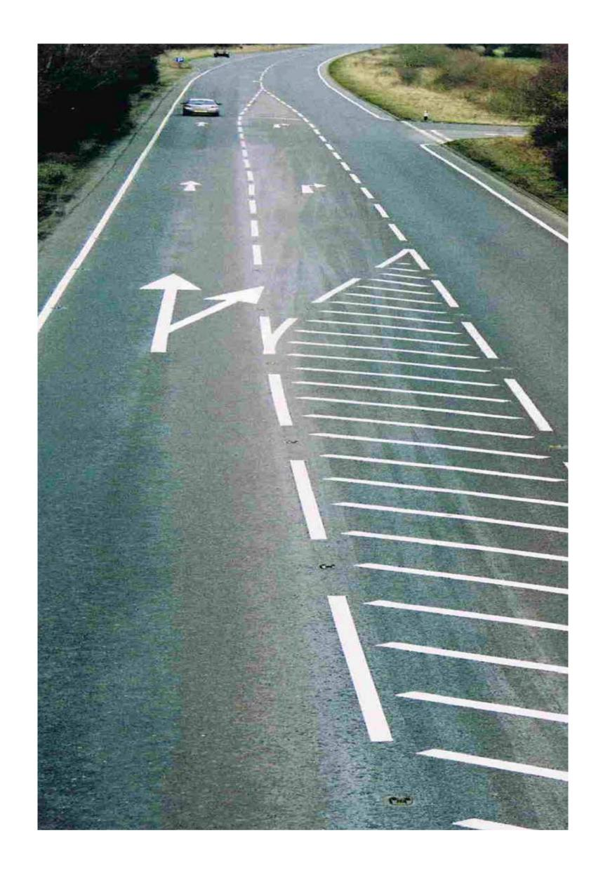
A ghost-island junction is a painted marking in the centre of the road. It allows a number of vehicles turning into the site to stop before turning, clear of the through-movement lanes. This will enable access for the properties located to the south west of the site.
